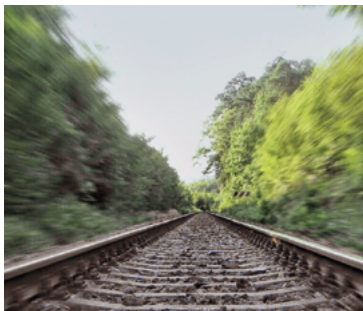
1 Track bed and gravel cleaning
